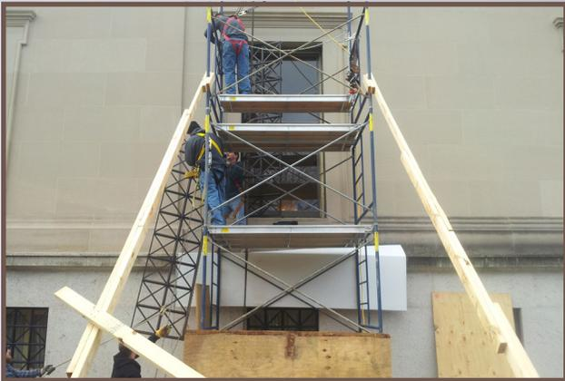
The refinished grilles were protected for transport. Each grille panel required three individuals to hoist them up on the scaffolding for reinstallation. The warmer brown color of the paint and grille complement the limestone exterior.
