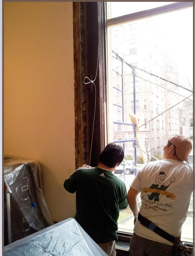
New cable was installed to carry the sash weights of the upper sash as the cable is not typically visible. Bronze sash chain is used for the lower sash weights where the chain is typically visible.
