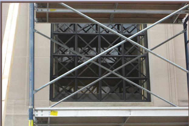
The grilles and sash are reinstalled with only the exterior brick mold to be painted. With the cold temperatures in March, the painting of the brick mold was deferred to warmer weather.
