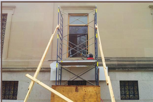
Scaffolding was installed on the S Street side of the building to allow access from the interior and exterior. Each window sash weighs almost 200 pounds, with 2 bronze grilles weighing closer to 400 pounds apiece.
