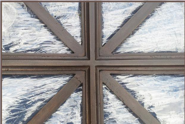
The detail of the grille is clearly evident with the refurbished finish. In addition to the oxidation process, lacquer was applied followed by a layer of wax. These sacrificial coatings provide protection against weathering.
