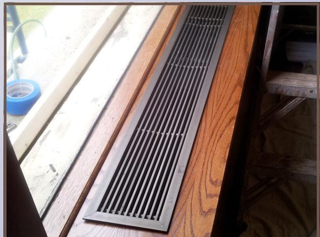
The sill of the fan coil unit (below the grille) was damaged by condensation. The existing grille was reinstalled in a new sill.
