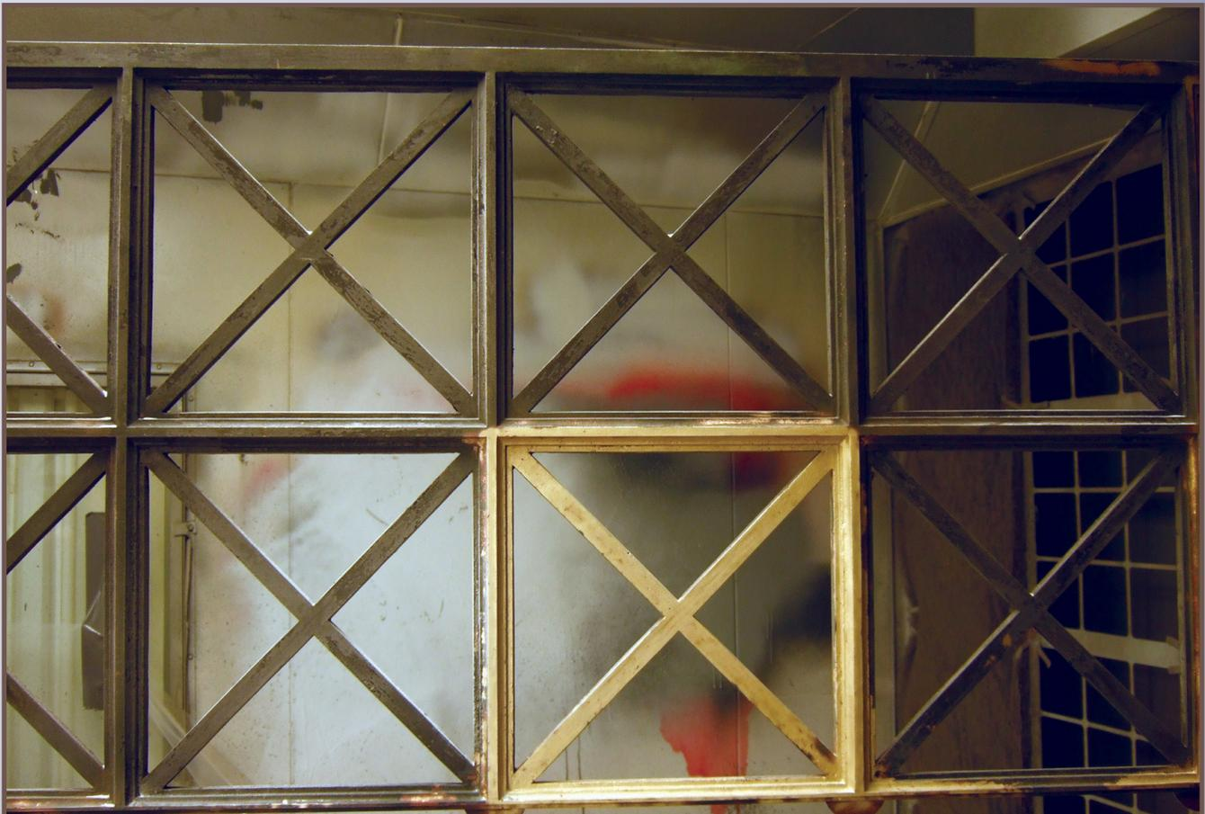
The existing grilles were over painted with paint at some point in the past. The team test multiple chemical strippers and media blast techniques to remove the paint without impacting the bronze grille. A medium grit glass bead was determined to be the most effective means.
