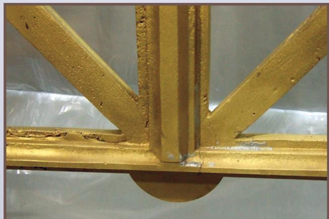
The bronze grilles were sand cast. In the cooling process the grilles shrank creating stress fractures in the finish. Some of these cracks were repaired with solder prior to application of the finish treatments. The sand casting process also revealed some "rough" edges.
