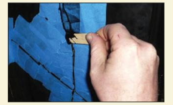
At either side of the doors to the Temple Room, cracks were found in the marble as a result of the earthquake. Fills were installed to the small crack losses in the black stone panels on either side of the door using a bulked epoxy colormatched to the stone. The surrounding areas were masked off to prevent any overruns of the patching material. The epoxy was then injected into the cracks and cleaned back with a razor after it had achieved an initial set.
