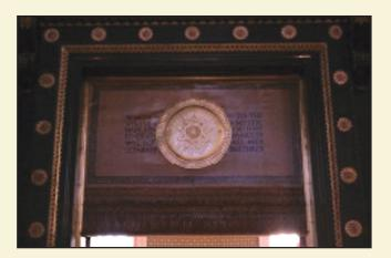
Areas of loss along the top left edge of the interior panel were patched with B-72 bulked with silicon microballoon and color-matched with mineral pigments. The fill was laid in with spatulas and trowelled to create an even surface. The color was adjusted with pigmented wax as needed.
