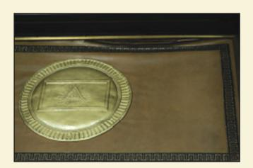
The August 2011 earthquake caused delamination of the leather panel at the door to the Temple Room. Sections of the bronze moldings were removed from the top and sides of the leather panels as needed to provide access for treatment by removing face screws.
