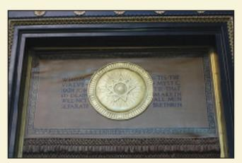
It was found that the leather had been directly applied to wood framing in-situ and was not installed on a separate panel. All leather was extremely desiccated and vulnerable to tearing. As such, it was decided to treat the panels in place rather than by removing them in order to reduce risk of introducing further damage.
