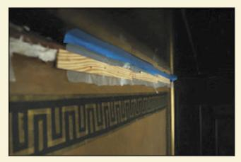
Linen strips were applied to the inner faces of the leather with BEVA gel adhesive to reinforce worn and brittle sections of the panel. The linen was extended a minimum of 2" beyond the panel edge and wood strips were tacked up to compress them while the adhesive set. Plastic sheeting was used to protect the leather during this work.
