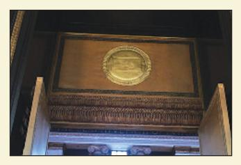
When the backings were dried, the leather panels were carefully stretched as much as possible without risking introducing additional tears and tacked with copper upholstery brads. It was possible to relay the exterior leather panel to its original position; however, the previous repairs—the nailer strip and a tack that had been added to the lower proper left edge at the tassels—had deformed and stretched the panel to the point where it did not allow it to fully return to the original contour.
