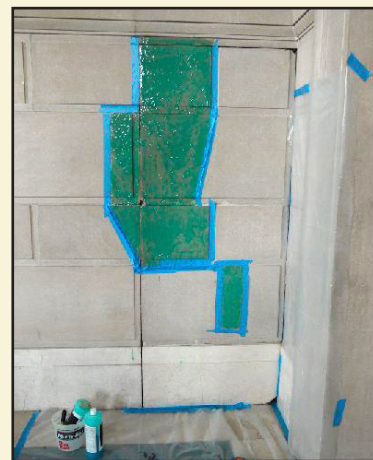
The gel was applied for a predetermined time.
