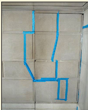
Area to be cleaned was taped off to limit spread of solutions to areas which were not to be cleaned.
