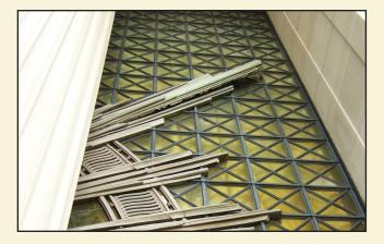
One of the rays from the "glory" on the West Elevation of the Temple Room became detached from the window as a result of the earthquake. Five panes of glass were also cracked or broken during this event. Conservators have reviewed the situation and proposed a methodology to reattach and stabilize the loose element.
