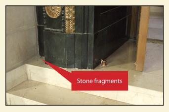
The stone fragments on the stairs outside the Temple Room are from a crack in the marble wall above which resulted from the earthquake.
