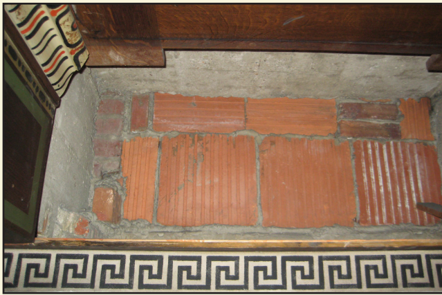
The second panel in the southeast corner was removed to reveal terracotta infill.
