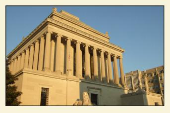
Where joints between the limestone were missing, new pointing mortar was installed. Once the overall building renovation is underway, the colonnade level and stepped roof will also be cleaned and restored.
