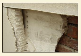
As the masons carefully cut out the joints of the stone panels to be replaced, they discovered that the surface was not stone but rather a mortar patch. Behind the mortar layer, was a later of stone, another layer of mortar, another later of stone mortared directly onto the brick back up wall which is inconsistent with the original drawings.
