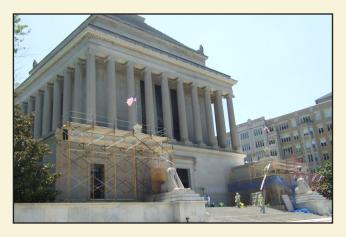
Scaffolding was temporarily installed on the north and south sides of the entrance to provide access to the stone walls.
