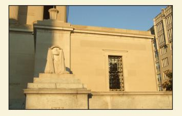
Following cleaning, the sphinx and walls are brighter with the heavy soiling removed as part of the cleaning. Malleable joint covers were installed on the top part of the wall to keep water from tracking down the joints.
