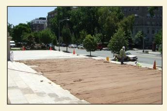
Damp burlap sheets where placed over the new mortar to allow the mortar to cure properly.
