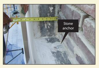
Once the non-original stones were removed, the original detail of the stone and brick was identified. Typically, the stone is six inches thick with a layer of mortar between stone and brick . Stone anchors were also identified in the construction of the wall.
