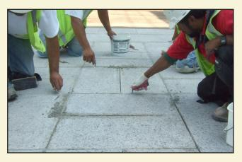
The joints between the stones on the plaza had deteriorated or were missing allowing water to migrate to the space below. After several mortar tests, the remaining material in the joints was removed and new mortar was installed.
