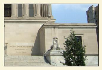
Before this current cleaning/restoration effort, heavy soiling was noted at the cornices and parapets of the west elevation. Additionally, four panels directly above the inscription on the building were inconsistent with the adjacent stone. Documentation indicated these panels were replaced with new in the last 25 years.
