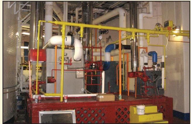
View of the boiler plant in the mechanical room. New energy efficient equipment will replace older boilers. New air handling units will be installed to heat and cool Temple Room, Atrium and Banquet Hall.
