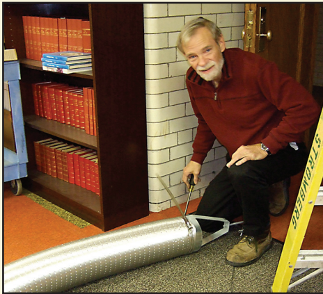
The existing duct work in the shafts was tested to confirm the ducts are sealed. The existing ducts were found to leak. The team is looking at alternative liners to insert in the ducts to transfer the air. Walter DePew of Stromberg Metal Works is installing flex duct in existing shafts as a test.
