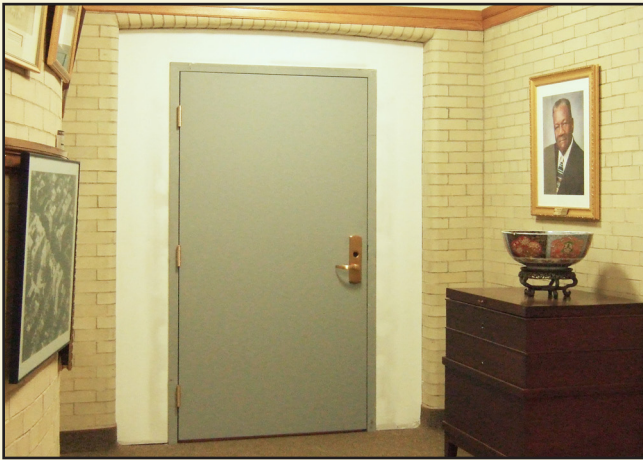
New doors were added at the basement level to separate the main stair from the basement level to minimize smoke migration should there be a fire event.
