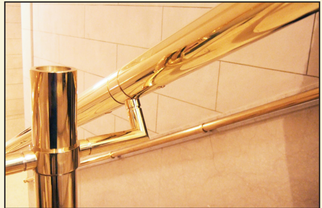
Close up of the center post and bracket supporting the railing. The detailing is similar to and respectful of Pope's detailing on the side rails.
