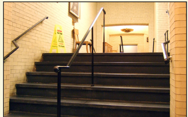
New center handrail added to the bottom run of stairs connecting the landing to the basement level. The design of the center rail is based upon the adjacent wall mounted rails.
