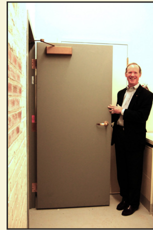
Architect Graham Davidson, FAIA holds open the new door isolating the mezzanine level from the NW stairs. The unpainted brick on the left of the photo is the location of the exploration of the brick wall thickness last summer.
