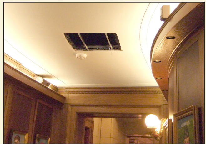
A hole was cut in the ceiling of the Portrait Gallery to allow installation of new fire alarm audio-visual device to alert visitors and staff to an emergency. Similar penetrations were made in the corridors outside the Burns and International Libraries.
