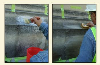
**Sample B:** The surface of the stone was pre-wet before the application of *Prosoco Light Duty Restoration Cleaner*. The solution was applied with a soft brush and allowed dwell for 10 minutes after which time a soft bristle brush was used to agitate the surface. The cleaner was allowed to remain on surface for an additional five minutes before being thoroughly rinsed.
