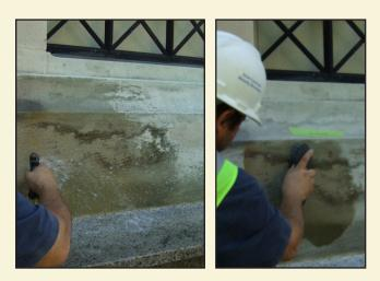
**Sample D:** *D/2 Biological Cleaner* by Cathedral Stone Products was sprayed onto the stone and allowed to remain for three minutes before the surface was agitated with a soft bristle brush. After a second application at five minutes, the entire sample area was thoroughly rinsed after a total dwell time of ten minutes.
