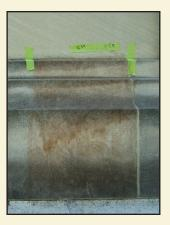
**Sample C:** The surface of the stone was dampened and the *masonRE B* cleaning solution by Cathedral Stone Products was applied with a soft brush. The *masonRE B* was allowed to remain on the surface for one hour before being thoroughly rinsed with water.
