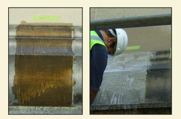
**Sample A:** *Deitrich 707X* was diluted one part cleaner to three parts water, applied with a soft brush and allowed to remain for one hour. After a thorough rinse *Deitrich 707N*, diluted one part solution to two parts water was applied and allowed to dwell for five minutes before being thoroughly rinsed.
