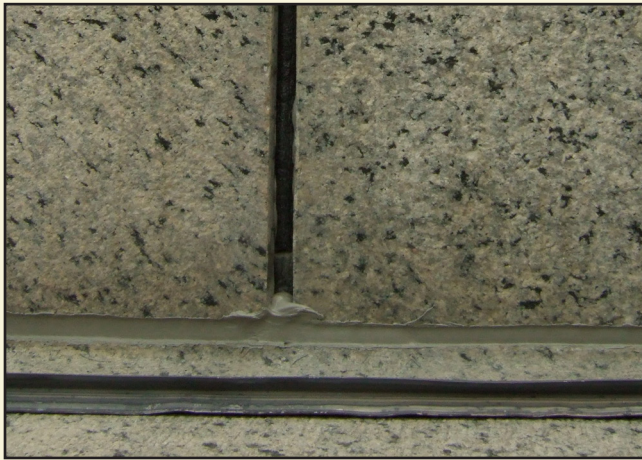
The existing, failed sealant joints are removed, new sealant and backer rod are installed in the open joints before the lead joint cover is installed.
