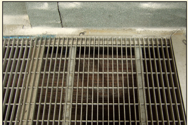
At the Colonnade roof, the replacement of deteriorated steel beams and installation of waterproofing in the air intake shafts and the new metal grates is complete.
