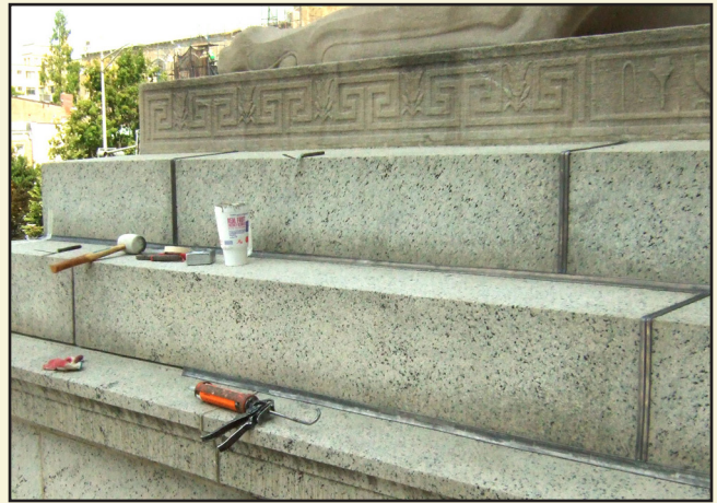
As part of the effort to minimize water infiltration into the building, the deteriorated sealant joints on the Sphinx pedestals are being replaced and protected with a lead cap.
