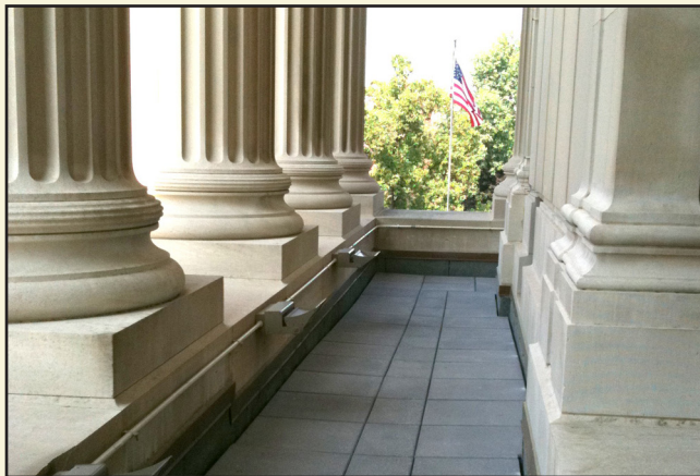
At the colonnade level, the existing failed roof membrane has been replaced with new roof membrane system with pavers.
