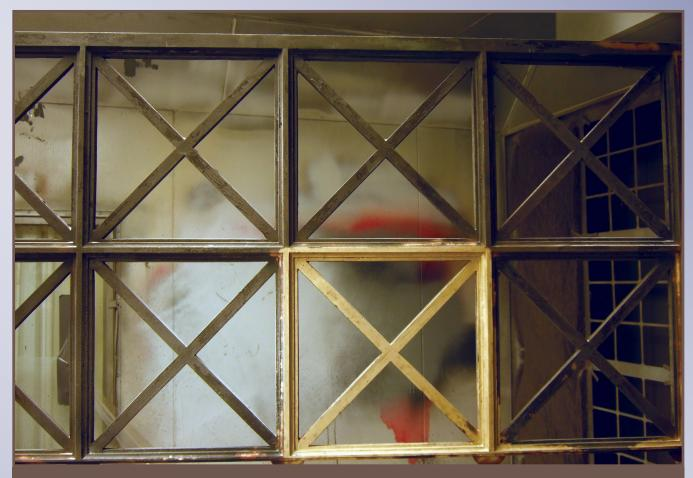
The existing grilles were over painted with paint at some point in the past. The team test multiple chemical strippers and media blast techniques to remove the paint without impacting the bronze grille. A medium grit glass bead was determined to be the most effective means.
