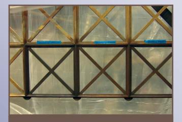
Three different levels of chemical patination were prepared to determine which treatment best matched the original finish. A clear coat will be applied over the treatment to stop the oxidation process and protect the grilles.
