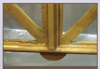
The bronze grilles were sand cast. In the cooling process the grilles shrank creating stress fractures in the finish. Some of these cracks were repaired with solder prior to application of the finish treatments. The sand casting process also revealed some "rough" edges.
