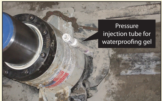
The waterproofing gel was pumped down the white tube to seal the casing. With the casing sealed and the piston in place, the "life jacket" will be installed, and the elevator cab will be reattached to the piston. The elevator passed inspection on April 22, 2011, and is back in service.
