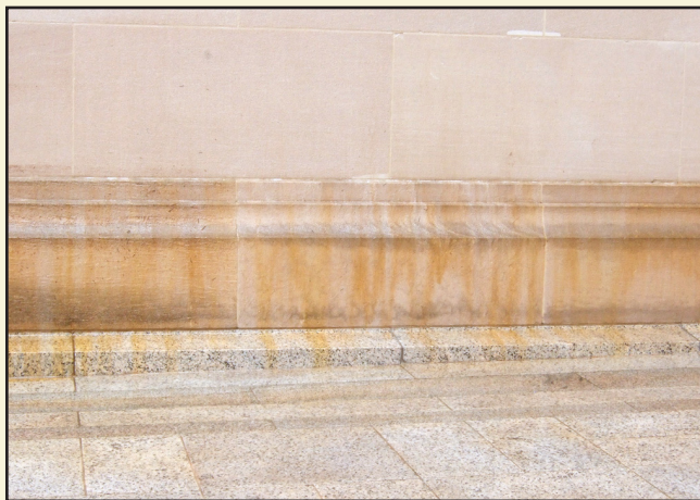
Using the Dietrich product tested in Fall 2010, the limestone at the entrance is being cleaned to remove the heavy soiling.
