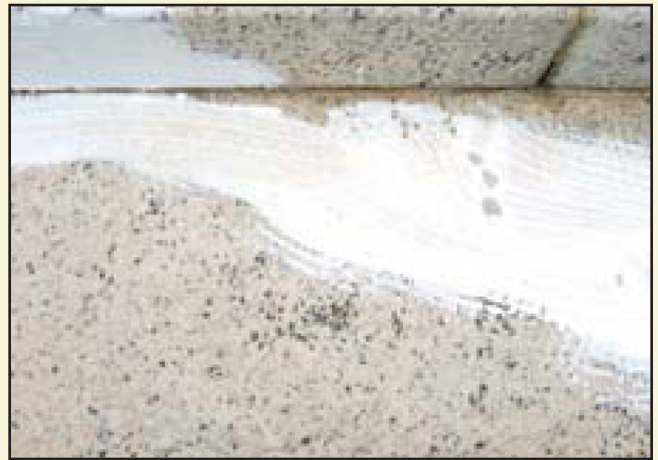
In locations where heavy soiling or petroleum products were found, a poulitice was used to “draw-out” the stain. The clear gel cleaner is allowed to dry to an opaque white before being removed and thoroughly rinsed.
