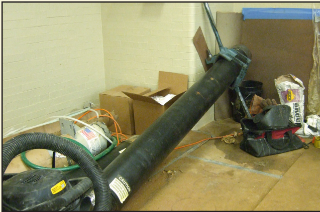
The new piston is being prepared to be hoisted into place in the shaft. Sections of the piston were welded together to create the overall length of almost 37 feet.
