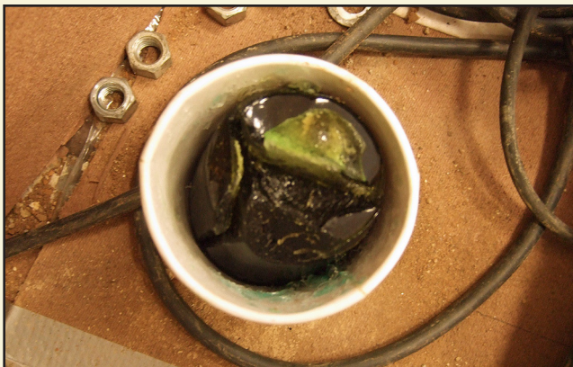
Due to the high water table around the House of the Temple, a waterproofing gel was pumped into the space between the casings to stop the water from migrating into the elevator pit. Each team of installers is assigned a different color so they know which "green" group worked on the House of the Temple.
