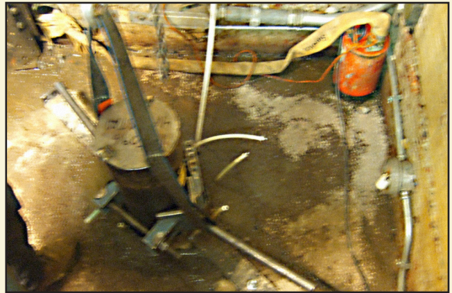
A section of the piston has been lowered into the casing in the elevator pit and is being aligned to ensure it is plumb.
