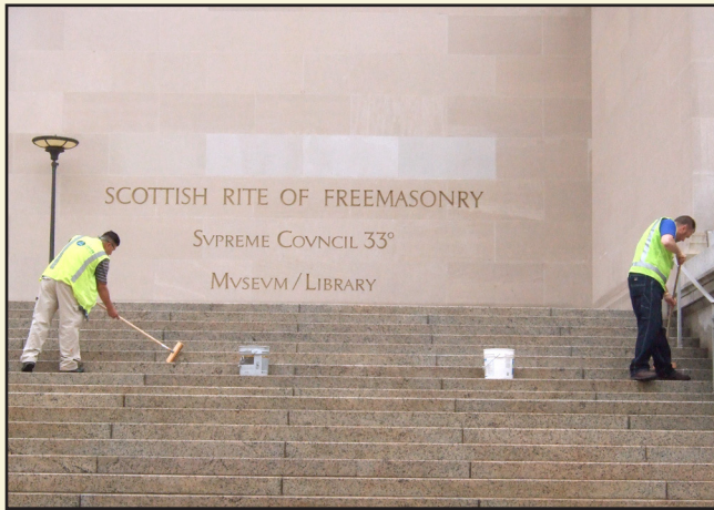
As part of the overall cleaning of the House of the Temple, the main entrance steps were cleaned using a light-duty restoration cleaner.
