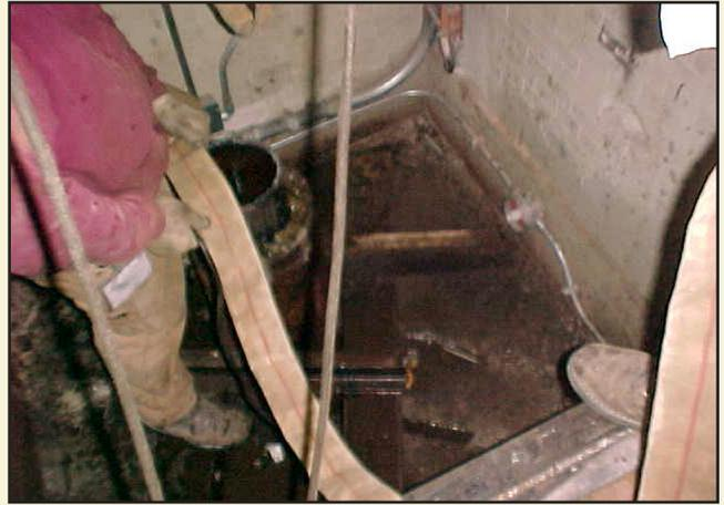
Hydraulic jacks were used to hoist the casing out of the hole.
