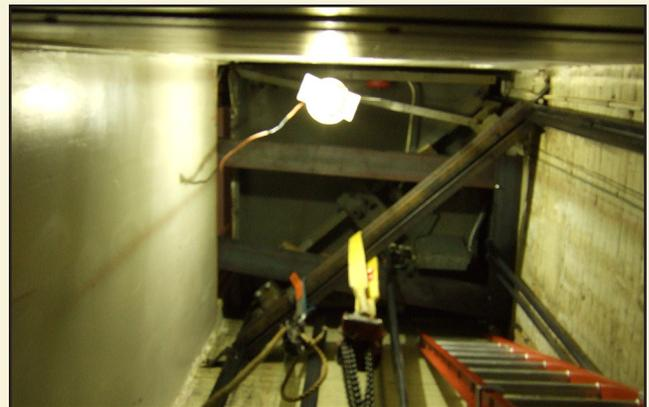
To allow the elevator jack to be removed, the elevator cab was raised to the parking lot level and temporarily supported on steel beams. Image is of the underside of the cab.
