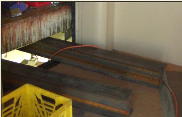
Steel beams temporarily support the elevator cab at the parking lot level.
