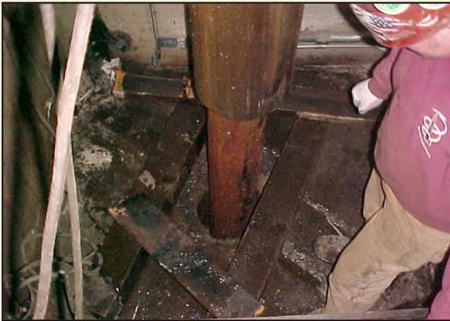
The casing and jack being removed from the hole. The old jack was only 11-feet into the ground. The new jack (to meet code) will be 31-feet into the ground.
