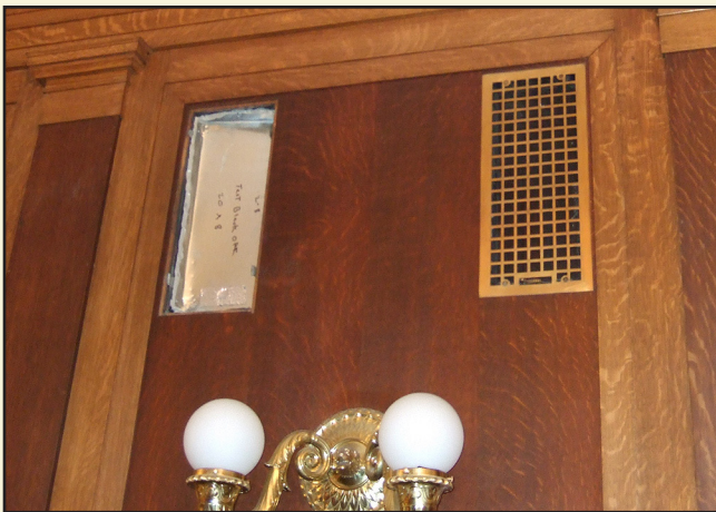
Ductwork providing air to the Burns (above) and International Libraries as well as the Executive Suites is being tested to determine if it can be reused as part of the renovation.
