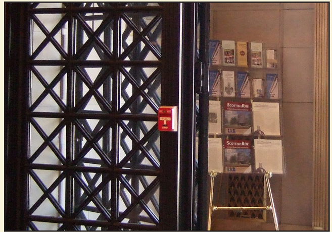
New fire alarm pull station added at the Main Entrance in the Atrium.
