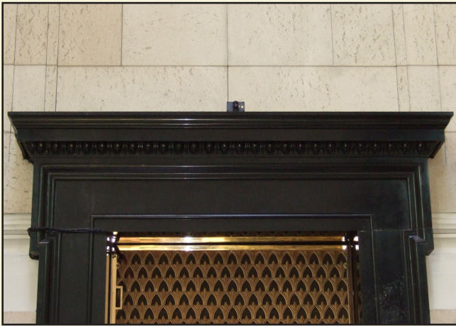
New video detection cameras in the Temple Room (above) and in the main stair use an algorithm to check the air for particles created when smoke or fire are present. The system will detect fires before flames are visible.
