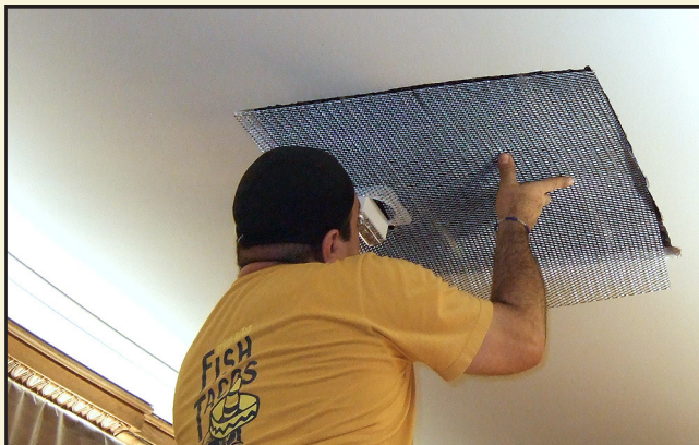
Installation of wire mesh to patch the ceiling penetrations where fire alarm devices were installed in the Portrait Gallery on the Ground Floor.
