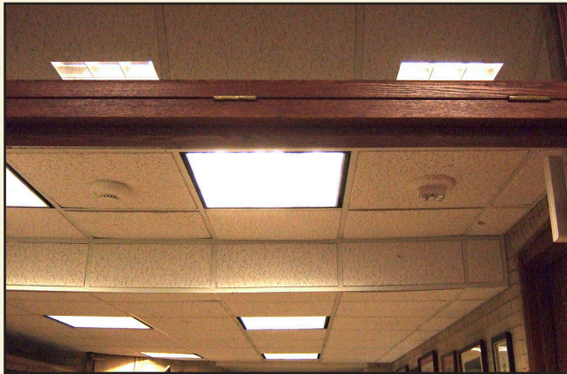
New smoke detector (to the left of the light) and fire alarm speaker/strobed (to the right of the light) added at the basement level.
