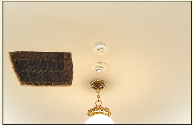
New smoke detector and fire alarm speaker/strobe added to the hall adjacent to the Americanism Exhibit. To facilitate installation of the new devices, a penetration was made into the plaster ceiling to install wiring and back boxes.
