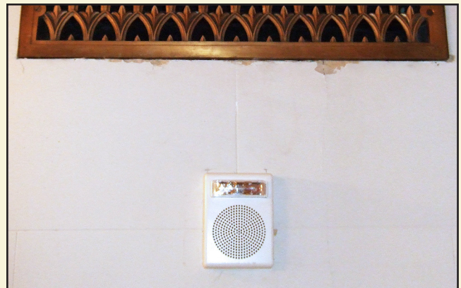
New fire alarm speaker/strobe installed in the Banquet Hall on the Ground Floor will alert guests and staff to a fire emergency within the building.
