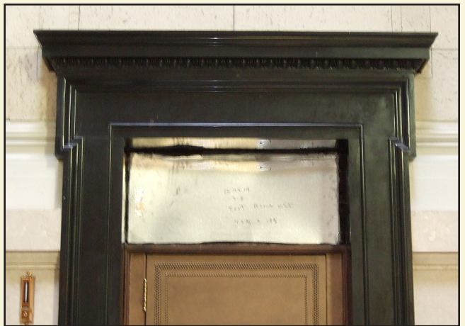
Ductwork providing air to the Temple Room is being tested to determine if it can be reused as part of the renovation.
