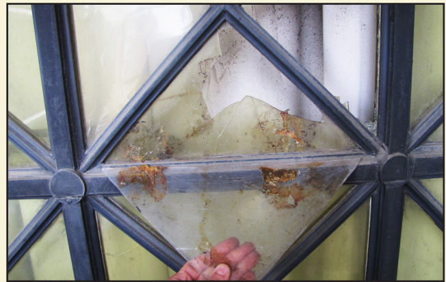
Example of Temple Room glazing which cracked during the earthquake. New glass is being fabricated and will be installed to make the window weather-tight. The yellow cast is accomplished by "painting" a glaze onto clear glass and then firing the glass in an oven. The glass is a deeper yellow at the bottom of the window transitioning to a light yellow at top of window.
